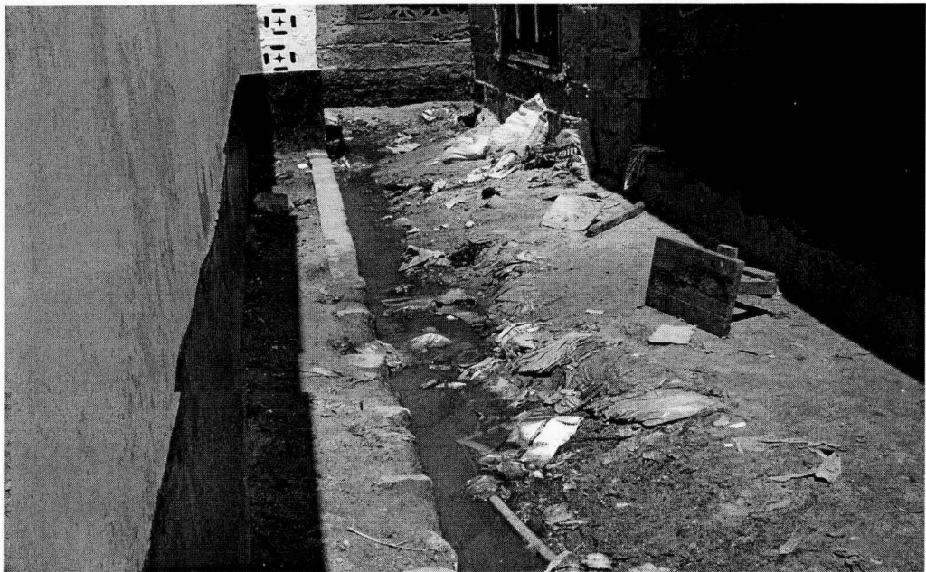
Photo.: situation in Hananasif area. Open drainage full of liquid and solid waste
